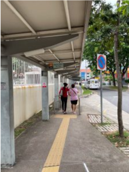
Sheltered walkway along Arumugam Road
