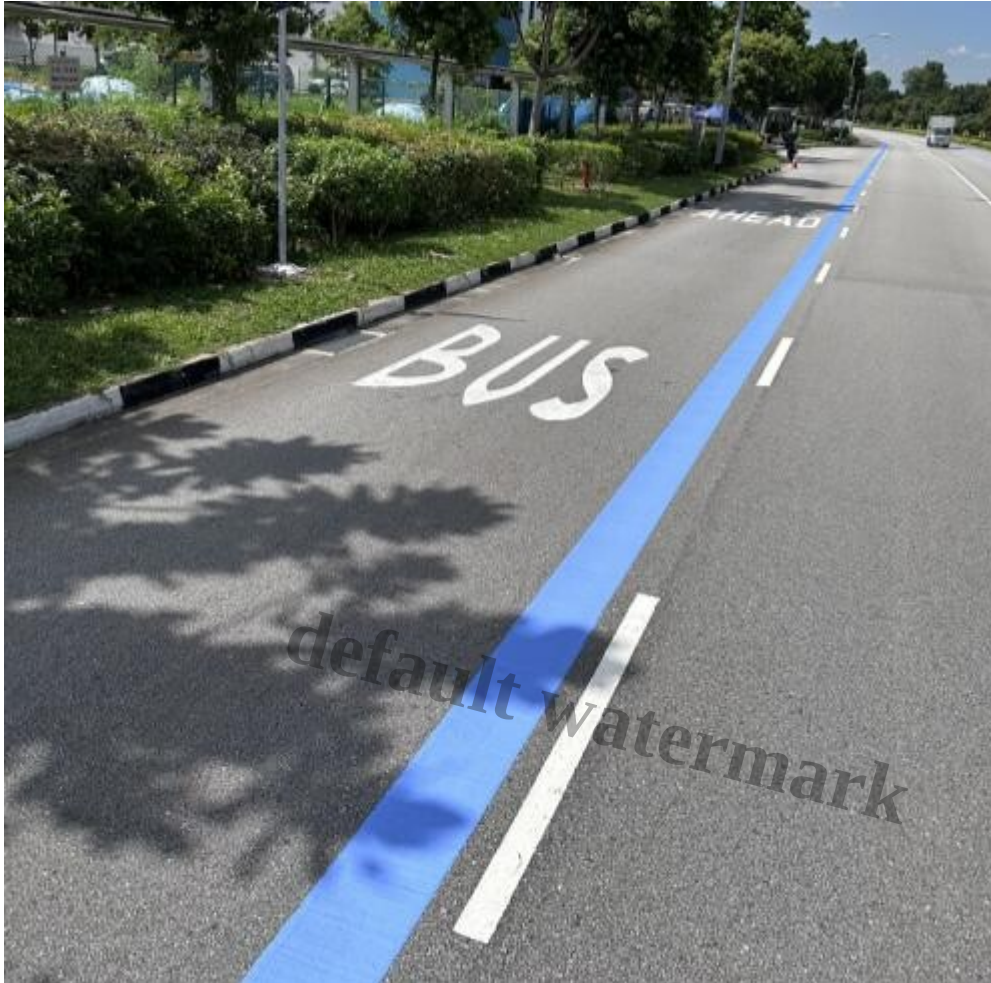
A solid blue line marks the cycling lane along the route. Photo: Land Transport Authority
