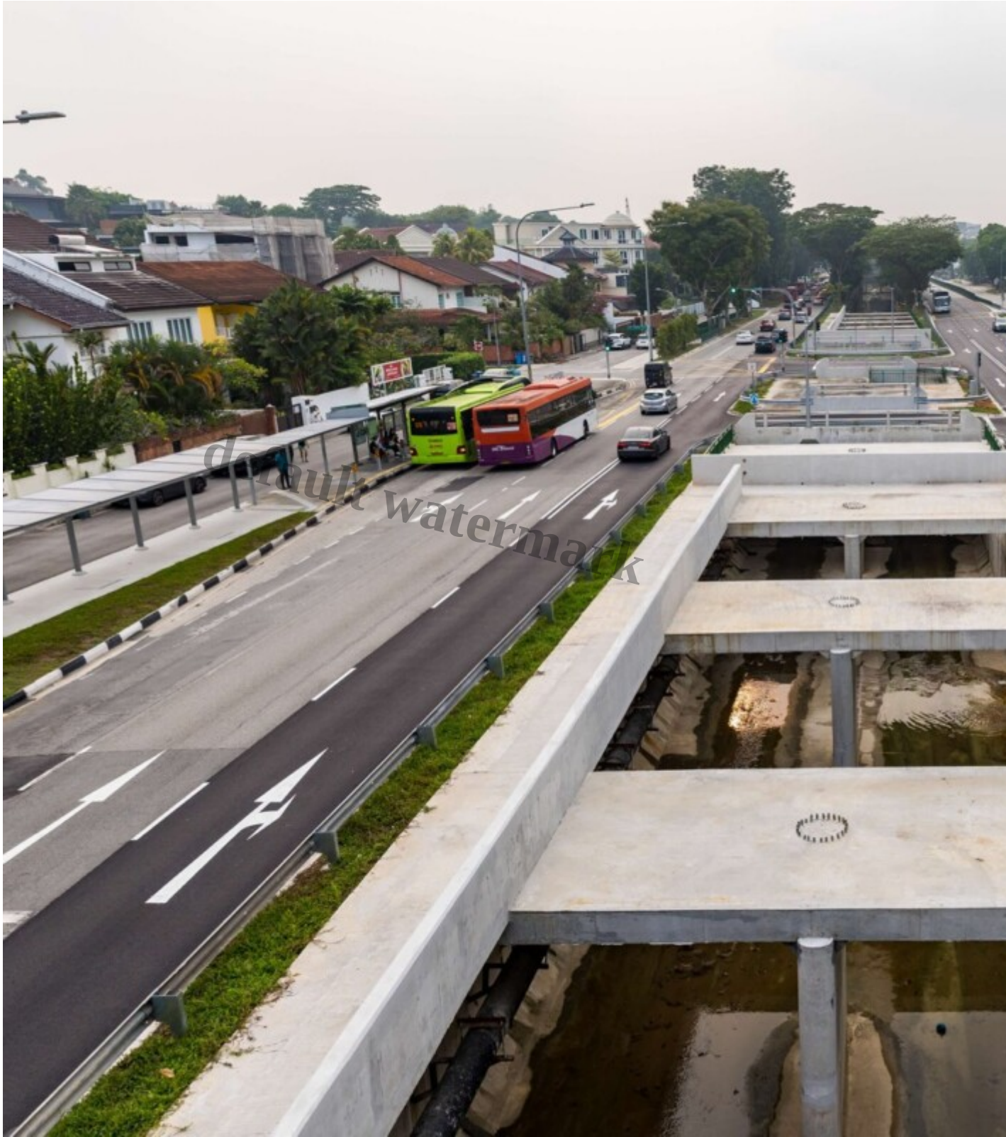
The upgraded Upper Bukit Timah Canal. Photo: PUB
