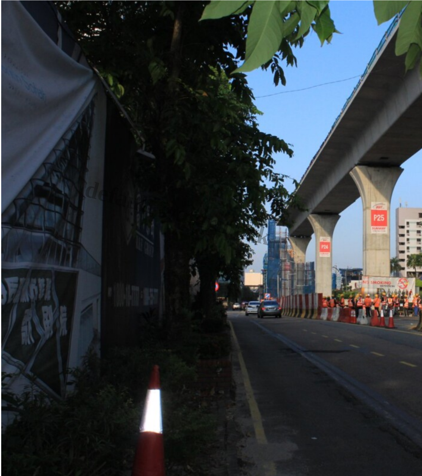
The 4km RTS Link viaduct under construction across the Straits of Johor. Photo: ZKang123 / Wikimedia Commons (CC BY-SA 4.0).
